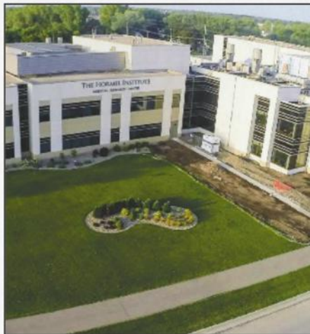
Harlan Johnsrud donated his drone photography talents to capture overhead construction of The Hormel Institute's expansion. His work will be featured throughout the Grand Opening ceremony and summer open houses to show the building growth and construction progress. Picture courtesy of Harlan L. Johnsrud.
